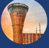
Goa International Airport, Mopa, Goa, India
